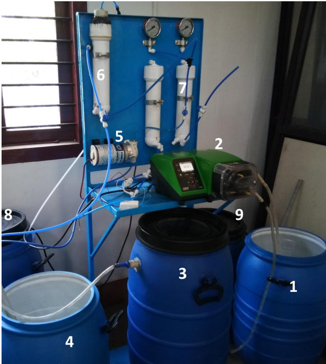
Figure 4.2. Photograph of the pilot-scale combined Bio-MF-RO unit for \text{ClO}_4^- treatment (1 - Perchlorate feed tank, 2- Pump (for bioreactor feed) 1, 3 – Anaerobic Fixed film Bioreactor (AFBR), 4 – Reactor effluent collection tank, 5 – Pump 2 (for MF and RO feed), 6 – Microfiltration unit (MF), 7 – Reverse Osmosis unit (RO), 8 – MF permeate collection tank, 9 – RO permeate collection tank)
