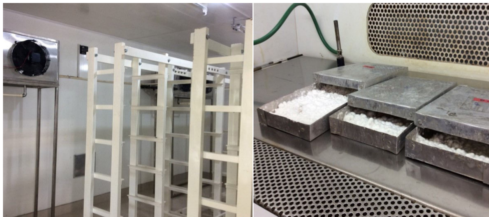
Koji Room (SSF chamber) showing steel racks for keeping trays and climate control system
